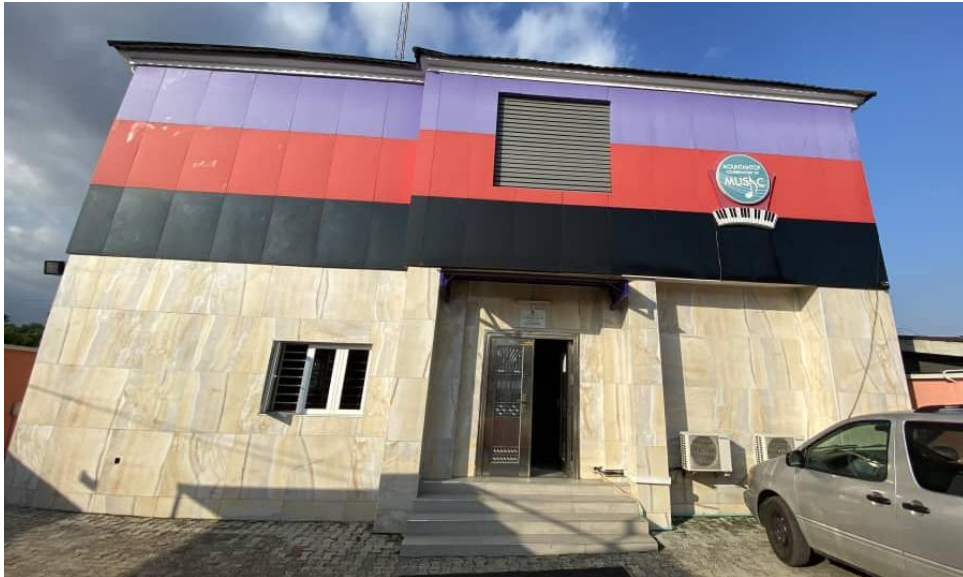
Photo 4: The front view of the Mountain Top Conservatory of Music
