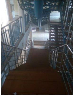
Fig 4: Stairwell, metro commercial plaza, FCT Abuja
