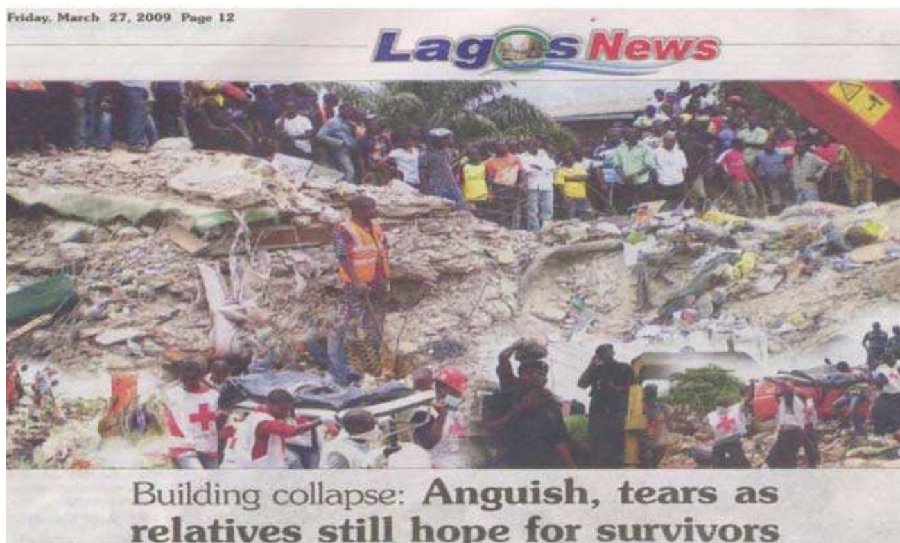
FIGURE 3. A Scene of Collapsed Building in Lagos (Source: The Nation, 27 March, 2009)
